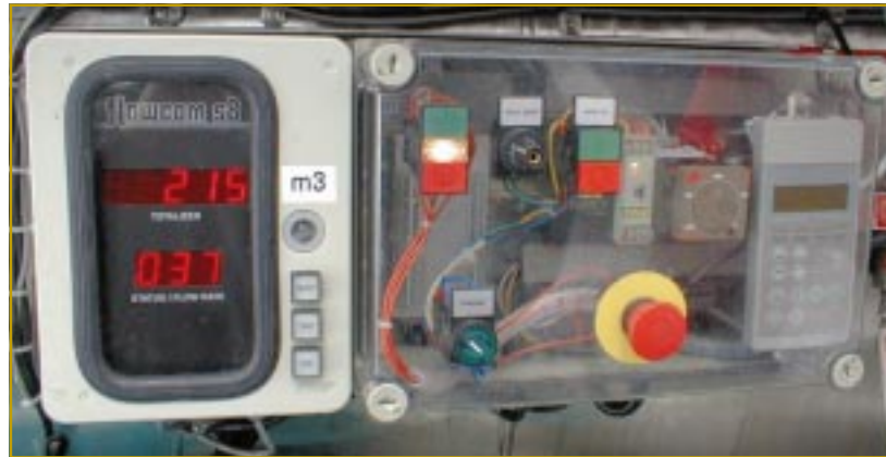
An ACD CRYO laser tank filling centrifugal pump system with a variable frequency drive installed on a cryogenic container.
