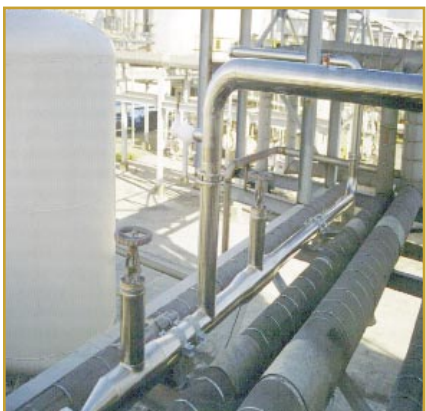
Pipeline installed in Taiwan.
