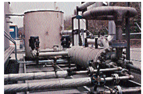
FIGURE 2—WCV Series back-up system with standing pilot natural gas water boiler.
