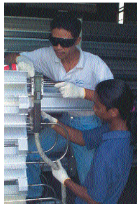
Cryoquip welders carry out orbital welding of stainless steel tubing on a high-pressure ambient vaporizer.
