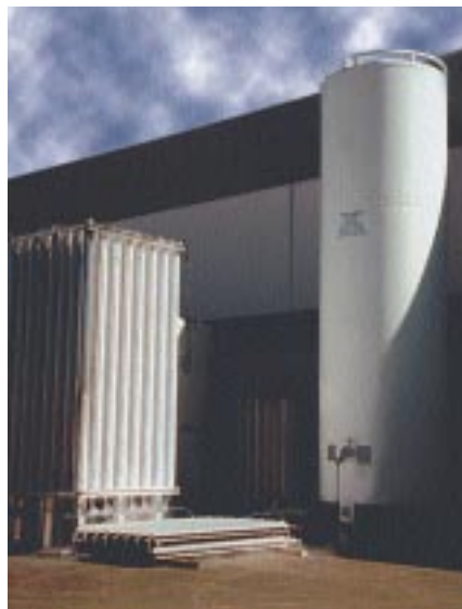
Providing the ice accumulation does not bridge the fin elements, the Cryoquip ambient air natural draft vaporizer will continue to function.
