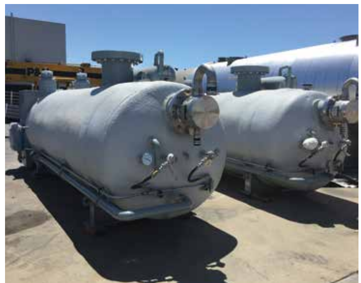
Figure 7 – Trailer mount natural gas fired water bath vaporizers
